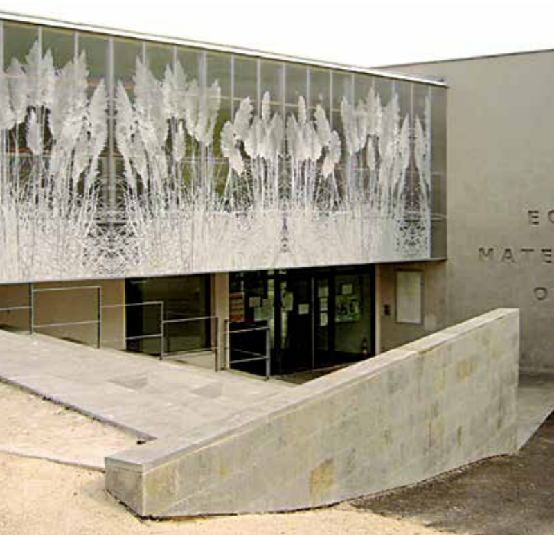
Oddo Nursery School, Marseille, France Glazing: Danpalon® Printed, 16mm Architect: Camille Richard Lenoble
